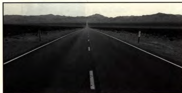
Highway 184 in Arizona
